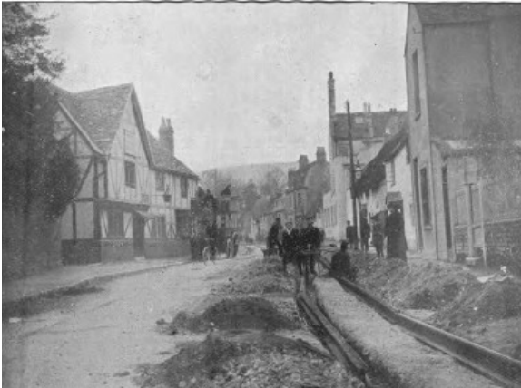
Laying the metals at Prestbury village
